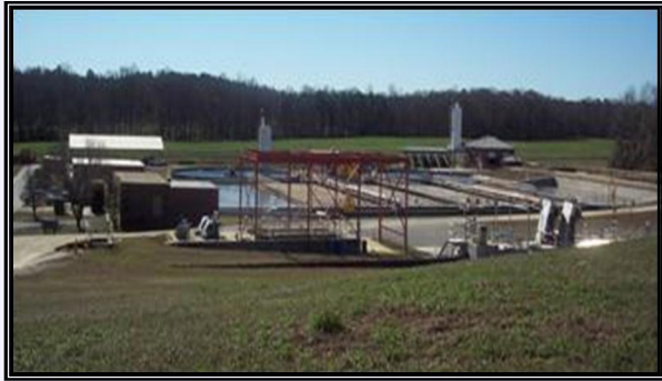
H.C. Morgan Water Pollution Control Facility (Auburn, AL)
